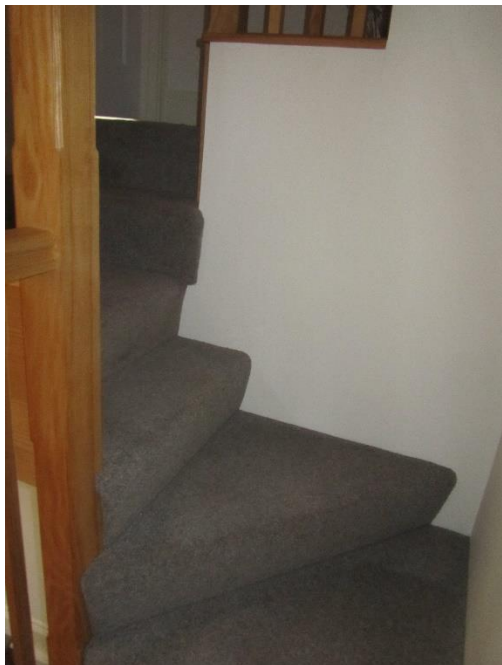
STAIRS TO THE LOOKOUT
