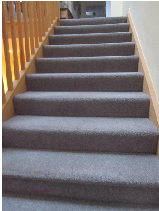
STAIRS TO FIRST FLOOR
